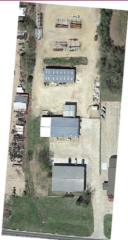
FORMER BLUESTEM ELECTRIC PROPERTY
